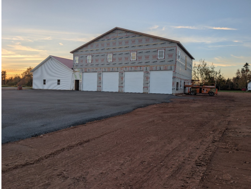
Front elevation: four new apparatus doors, wrapped exterior and paved apron.
