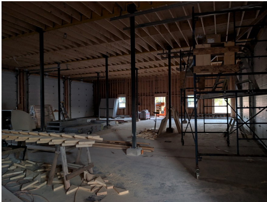
Interior: structural steel, overhead framing and ongoing partition construction.
